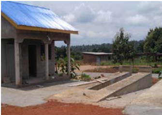
Work on Car Washing Bay for the Church and Community
